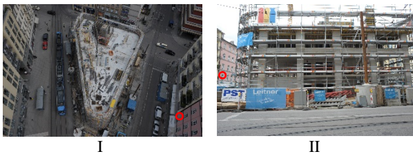
Figure 5. Example for two images taken on the construction site. Image I is taken from the crane. The red circles show a control point.
